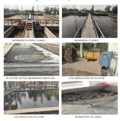
FIGURE 3.4: Primary and Secondary treatment
